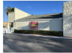
500 sq/ft Awning will be removed
