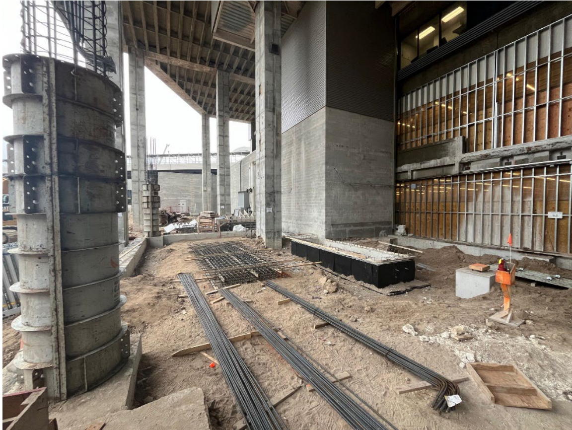
East Side Grade beams and Columns
